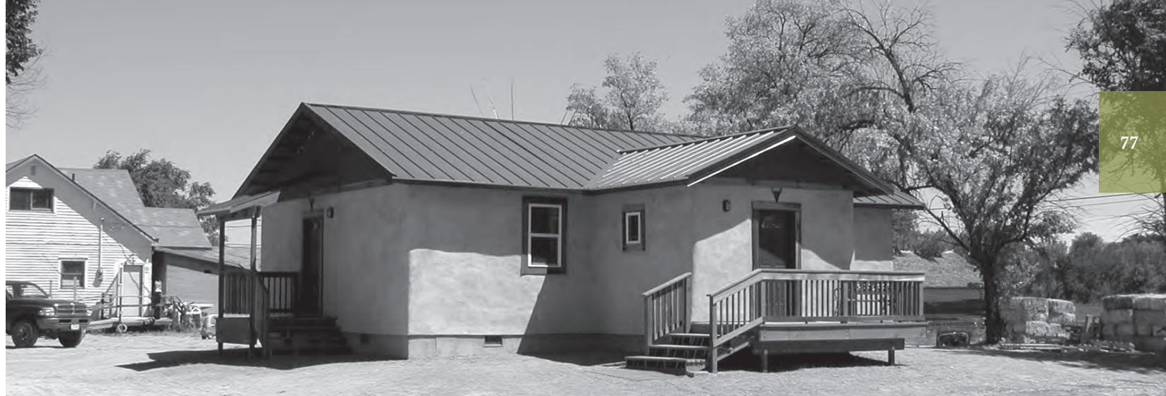
Study Hall for the Crow Nation Reservation, Montana, built after four students won a National Science Foundation contest for their idea to build affordable housing using straw-bale construction.
