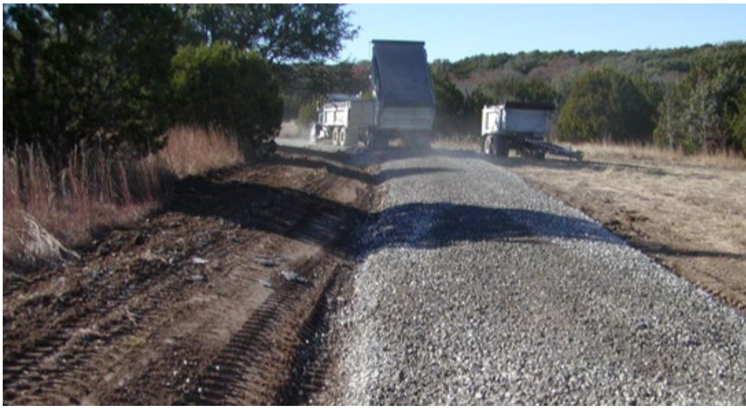
Laying down aggregate road base
