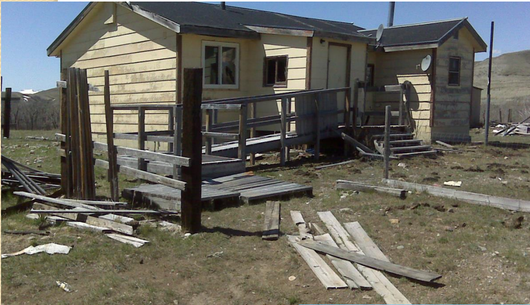
Blackfeet – Renovation (before)
