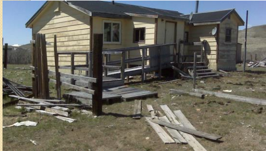
Blackfeet – Renovation (before)
